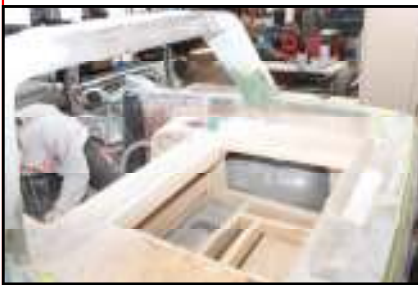
The back roof removed, and work is progressing on the fiberglass of the sun deck, complete with a hidden refrigerator.
